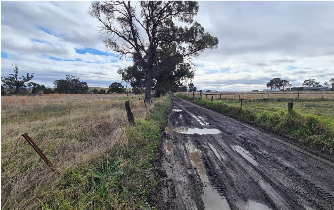
Figure 20 Exposure along farm track
