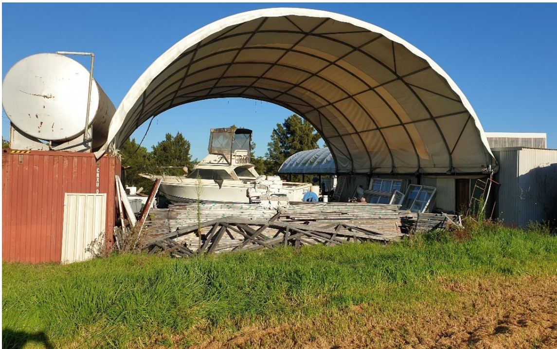
Figure 17 Constructed shelter positioned at the centre of the property
