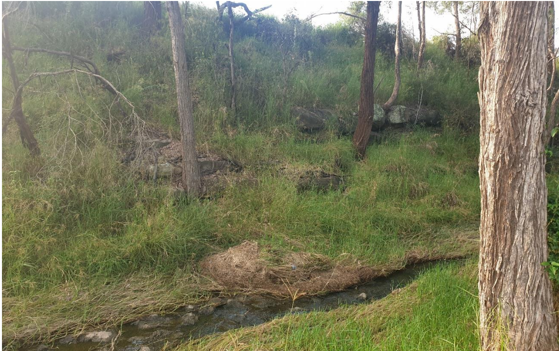
Figure 32 Embankment constructed for Hume Motorway
