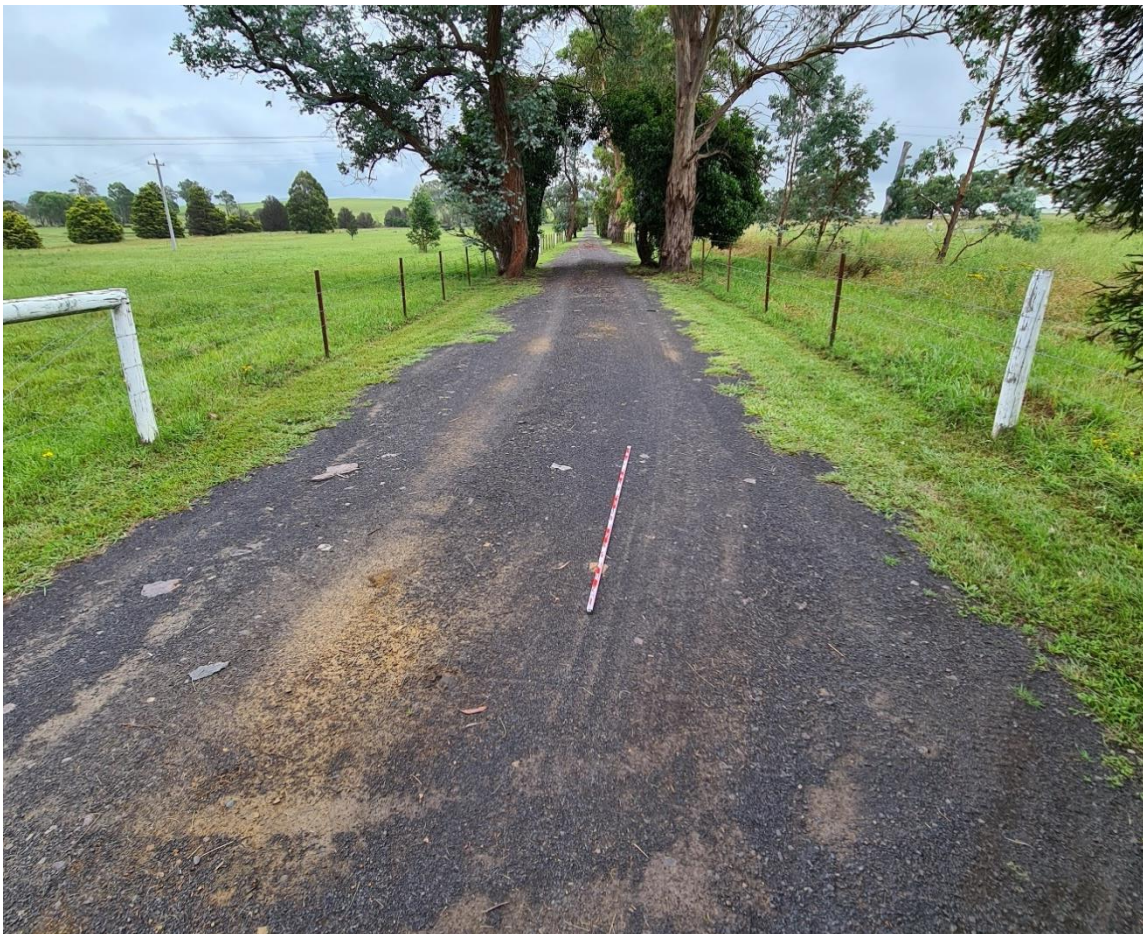
Figure 4 Gravel driveway, view north
